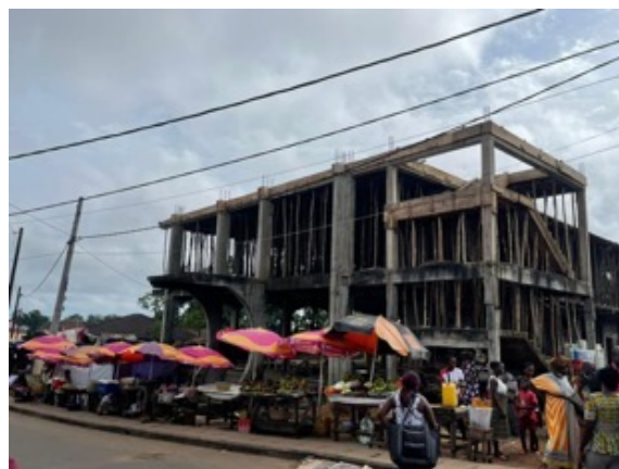
Wilberforce Market under construction
