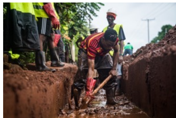
Drainage clearing exercise by community volunteers
